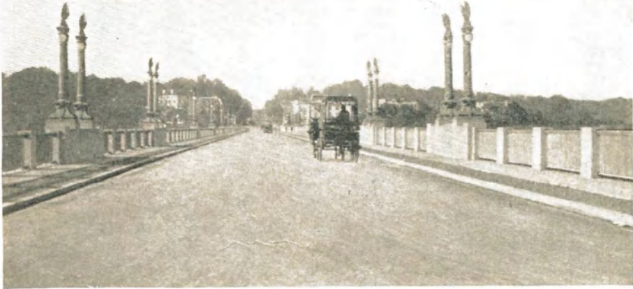
Connecticut Avenue Bridge, Washington, D. C. Roadway Built with Tarvia X.
